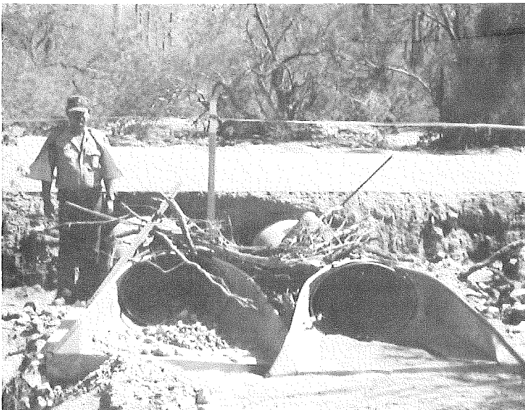
Photo on right: Erosion that occurred where roads crossed washes. A rock foundation, probably built by W.P.A. crews during the depression of the 1930s, was exposed and partially removed by the runoff. Photo on left: Debris-laden water, flowing toward the foreground, plugged upstream end of corrugated pipes. Water then flowed across road, undermined the pavement, and washed away fill material at the downstream end.
